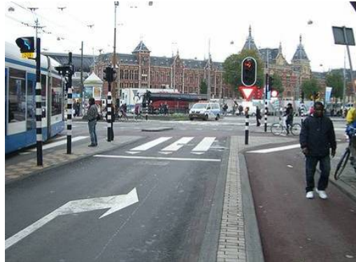
A channelized right turn puts the cyclist onto the cross-street
