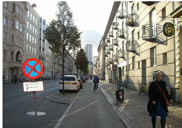
Figure 1. Cycle track in Amsterdam with on-street parking and planted curb extensions
