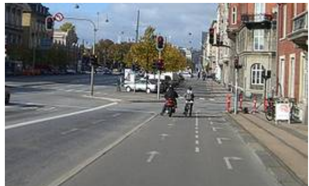
Figure 13. Straight and right turn (extended cycle stacking lane) at intersection, Copenhagen
