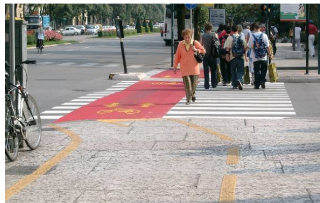
Figure 9. Bike lane marking continues through the intersection
