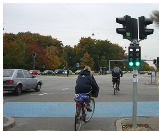
Figure 12. Bike-specific signals are small and placed on the near-side of traffic
