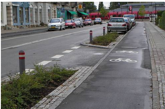
Figure 6. Bicycle markings at a driveway crossing clearly designate that bicyclists have right-of-way
