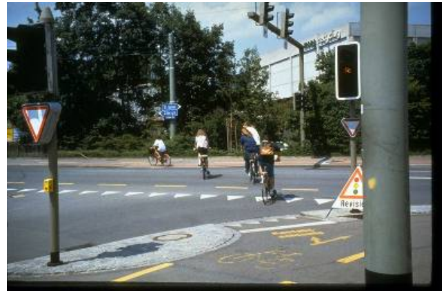
Figure 14. Left-turn from a cycle track on the right via bicycle-signal phase in Winterthur, Switzerland
