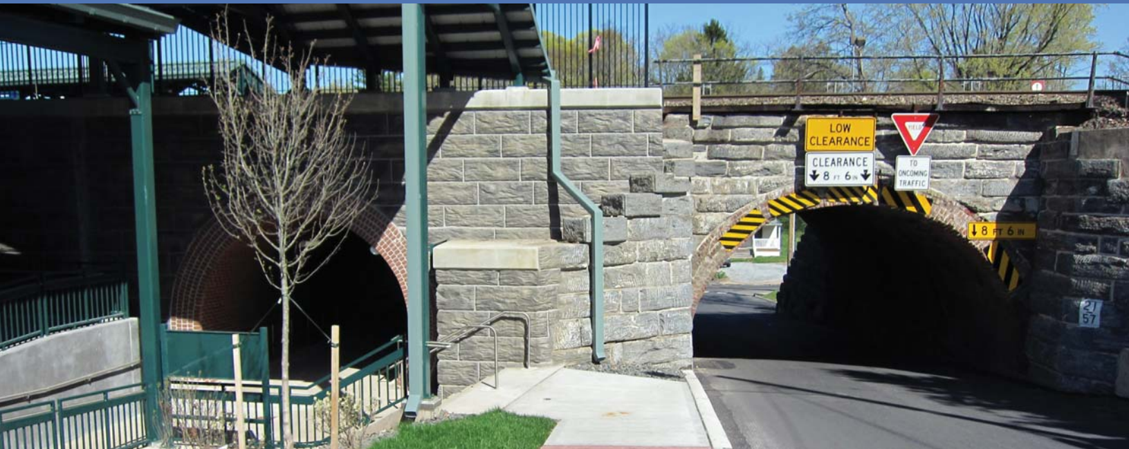
Pedestrian and handicapped access, in addition to parking have been improved at the Malvern station of the Paoli—Thorndale rail line recently.
