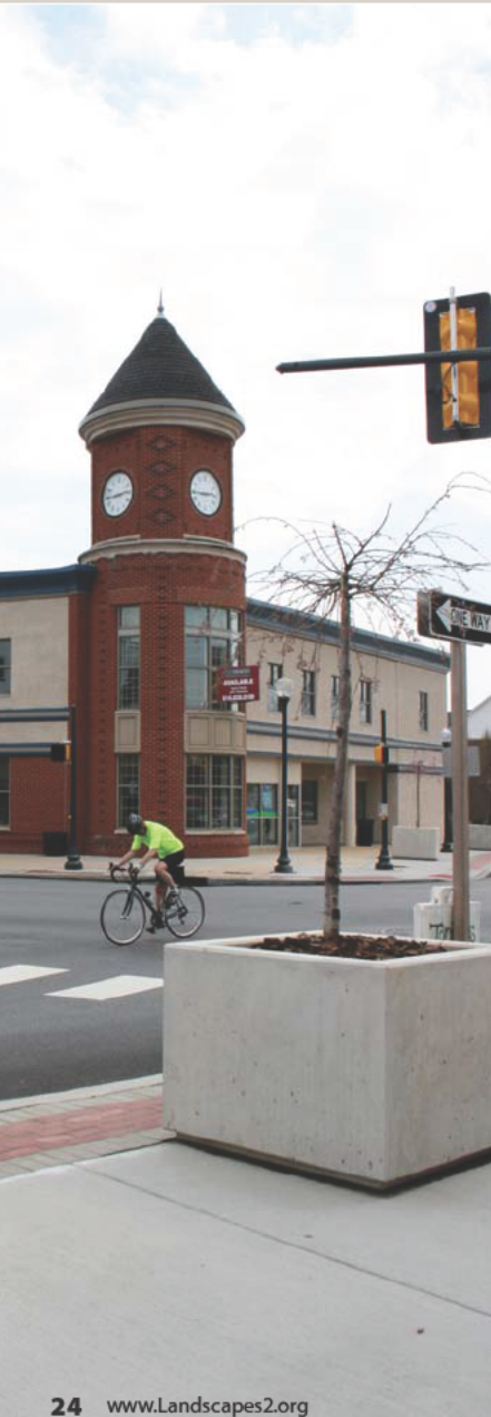
Funding for streetscape and signal improvements in Coatesville and Downingtown (shown) were provided through two DVRPC funding programs.
