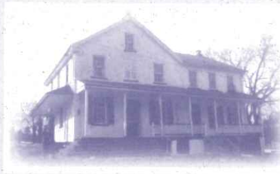
General store on site of 1786 inn
