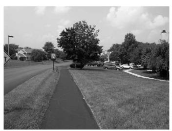
Macadam is preferred for paths since it has lower maintenance cost and is less susceptible to stormwater erosion.
