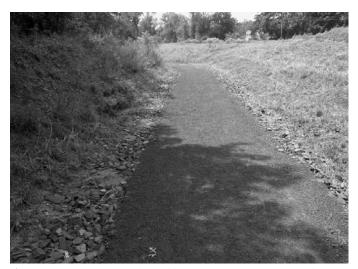
This compacted gravel trail has a coarse stone curb to protect it from stormwater erosion.
