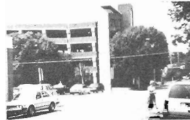
-1.90 Parking Garage Slide #52
