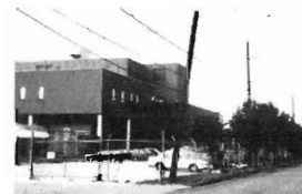
-3.69 Industrial Facility Slide #67
