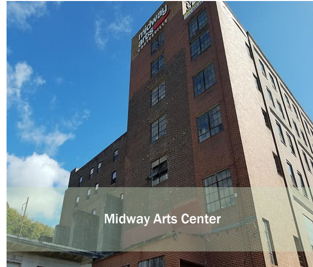
View of Midway Arts Center from Lincoln Highway
