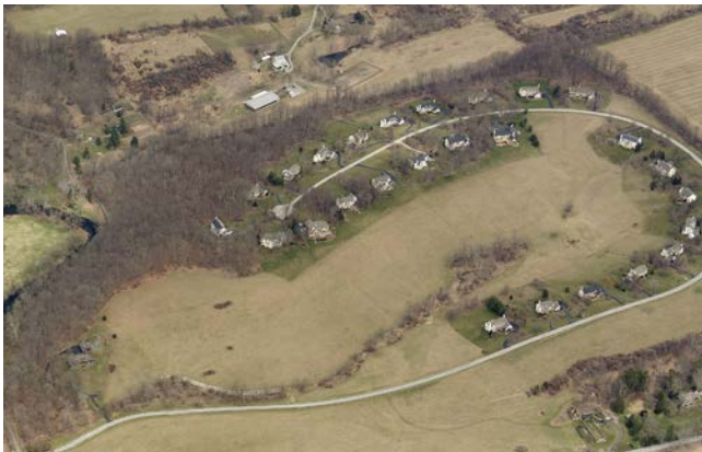
At Parke Farm in East Bradford Township, 34 single-family homes on 2-acre lots are surrounded by 200 acres of protected open space. The topography, existing woodland, preserved hedgerows, and thoughtful layout of this development provide an effective screen to adjacent uses.
