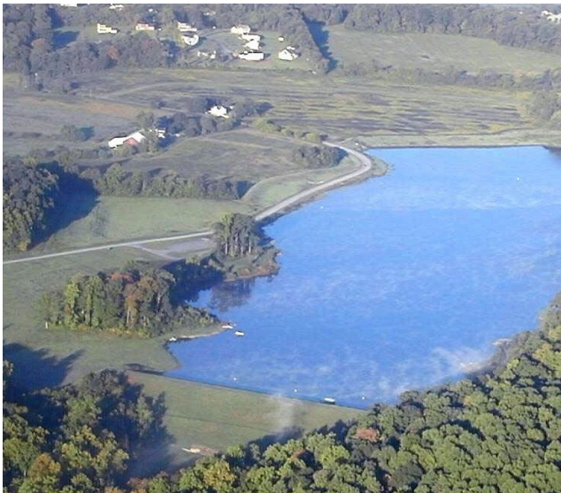
West Caln Township, where Chambers Lake is located, enacted an ordinance in 2021 establishing a sewer management program for individual and community on-lot disposal systems.
