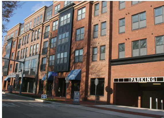
Chestnut Square Apartments, West Chester Borough has two levels of underground parking (1.5+ spaces/du)
