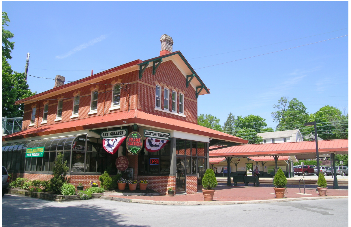
Berwyn Train Station serves as a focal-point to the village.
